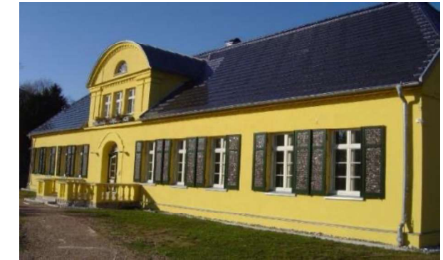
Historic renovation with PV-shutters (by Astrid Schneider) and PV-roof tiles. Solar Centre MV – by SIM e.V.
