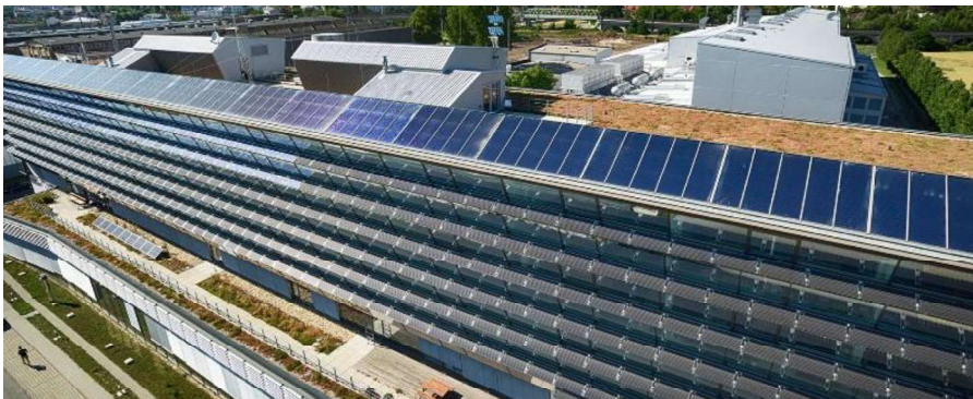
PV-Façade and solar thermal collectors at Energybase office Building in Vienna, project by AIT-Austrian Institute of Technology, Architect Ursula Schneider
