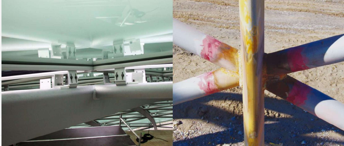
Hangar 8, Salzburg © Bollinger + Grohmann Ingenieure, Frankfurt
