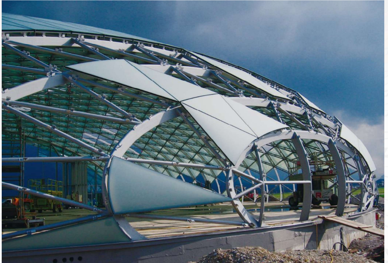
Hangar 8, Salzburg © Bollinger + Grohmann Ingenieure, Frankfurt
